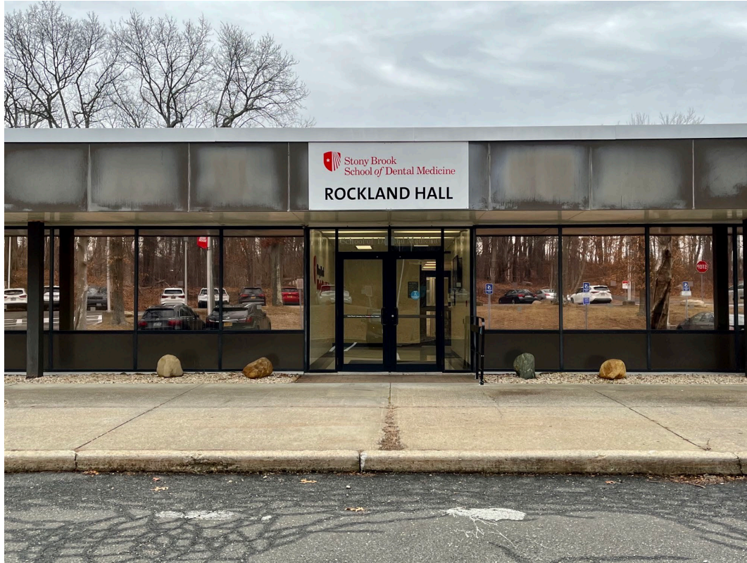
ADA entrance and improved curbing
