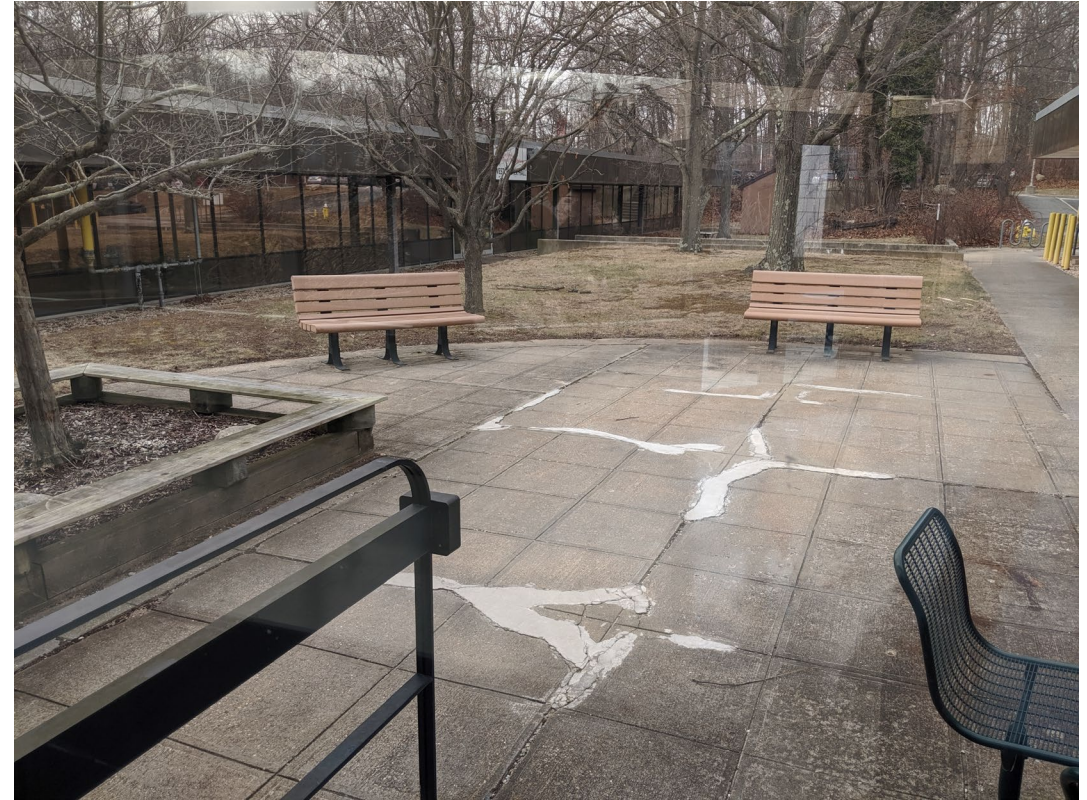
Courtyard – new pavement and furniture
